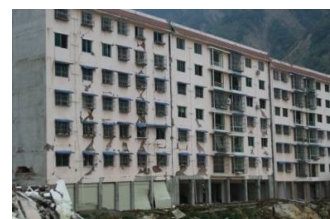
c) Moderate in-plane damage
